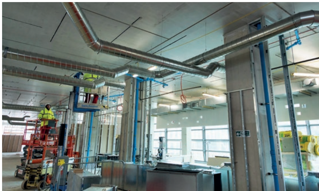
Above: Work starts inside as concrete frames are completed.
